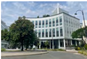
Rueil Malmaison Headquarter (Ile-de-France - France) 350 people
